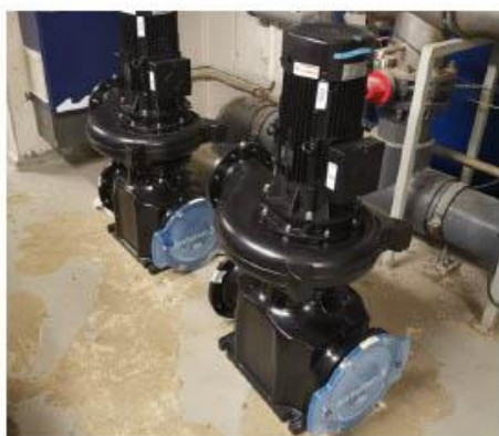
The new swimming pool circulation pumps
