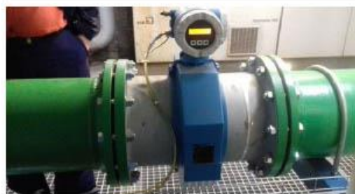
Flow meter installed following WaterWatt project at DEW
